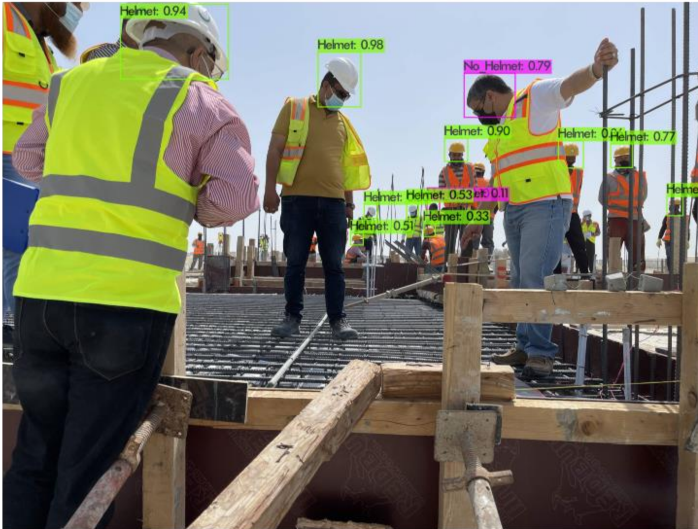
Figure 28: Site inspection (Housing Foundation) in Wadi Al Sail Housing Project
